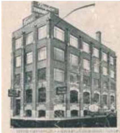
Office and manufacturing plant, Church St, Toronto 1934
